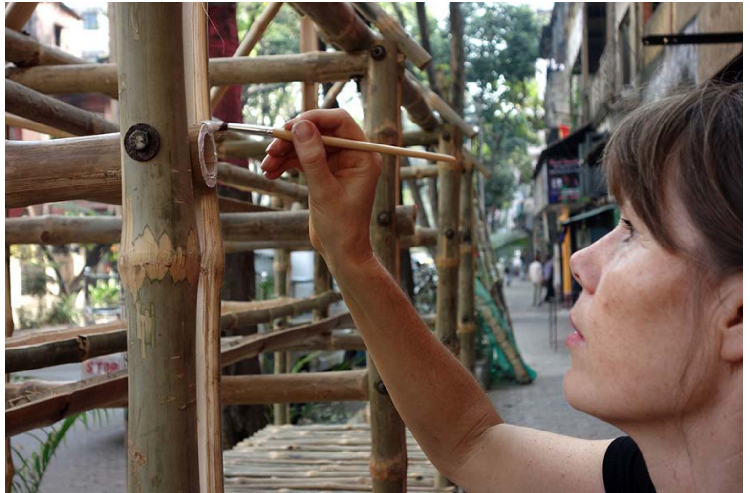
Painting white ends on the bamboo Palki
