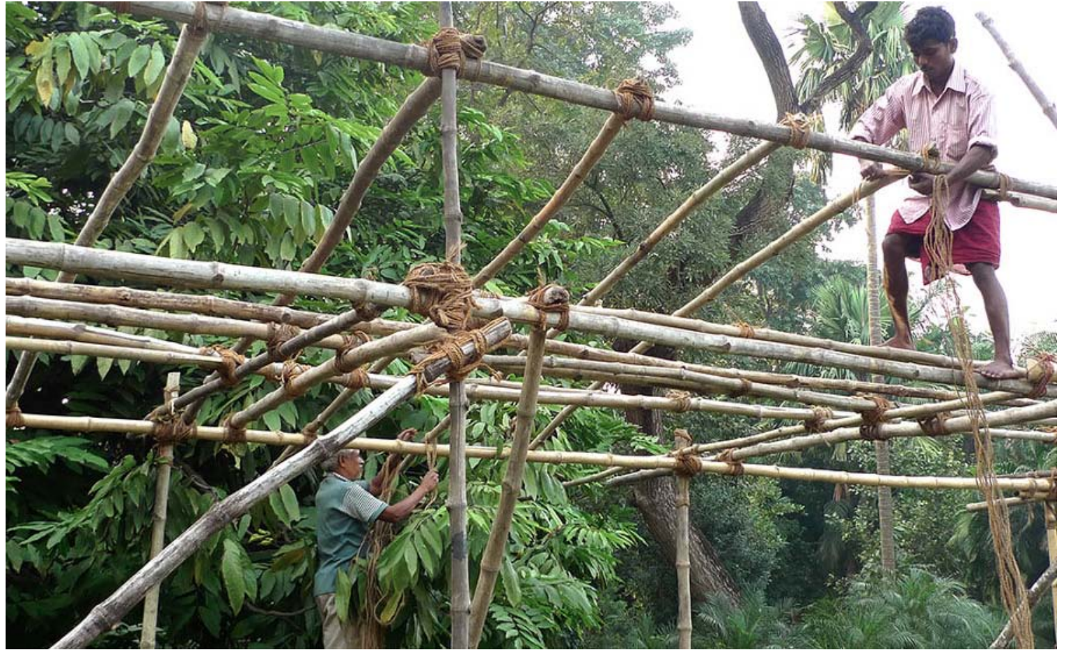
Study of binding techniques with coconut fibres.
